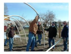
The hoop house ribs are made from 20 foot lengths of two inch schedule 40 PVC pipe. This allows for a 12 foot wide greenhouse with a center height of about 6.5 feet. Research by Mr. Jimenez indicates that PVC pipe with a diameter smaller than two inches is not advisable as high winds and snow loads will significantly decrease the structures lifespan. One end of the PVC pipe is placed over the previously placed rebar and bent so the other end can be fitted onto rebar stake on the opposite side.
