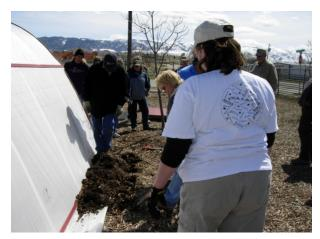
After the plastic has been attached to the hoop house frame, dirt is piled on the excess plastic to help protect it from the wind. This seals up the bottom and adds weight.
